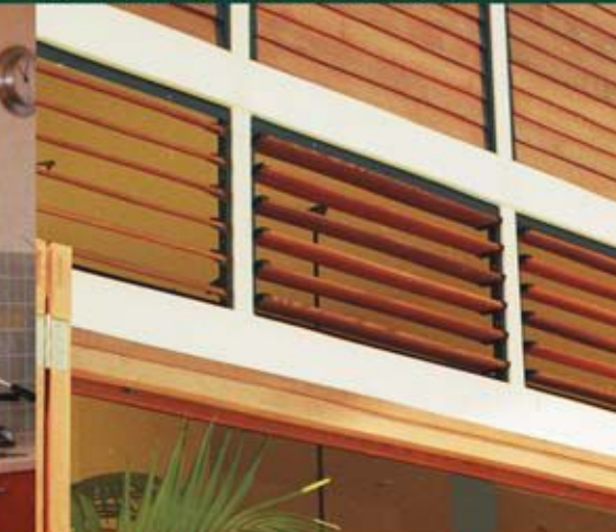
Timber Louvre Assembly
